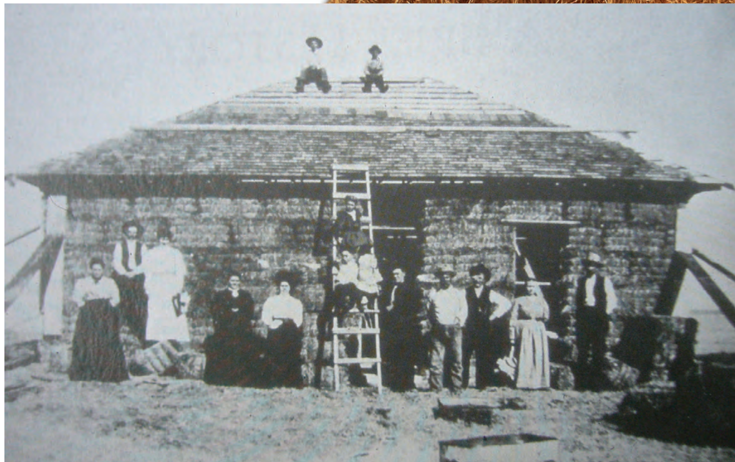
Fig.1. Simonton House. Nebraska—1908
