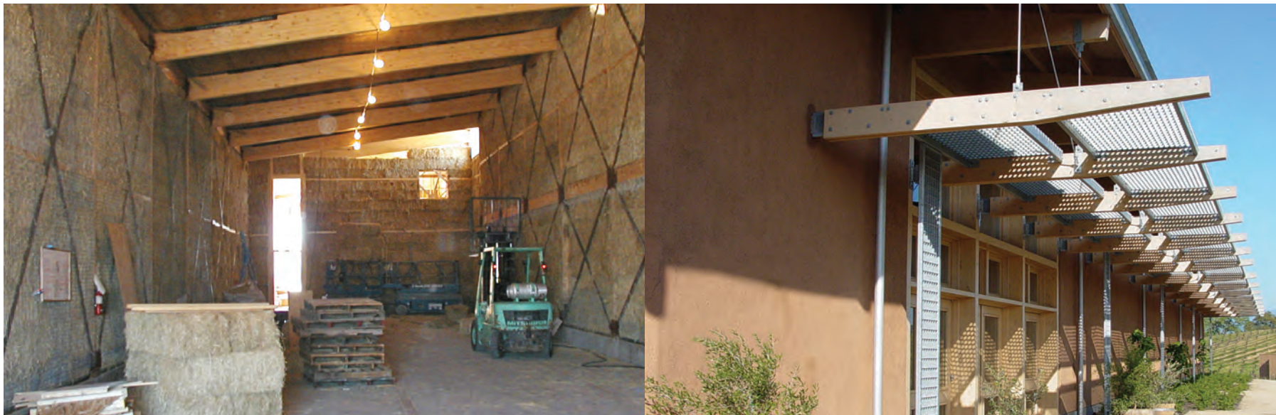
Fig. 2. A contemporary strawbale building. Ridge Winery, California, 2002. Interior before plaster, exterior finished. Freebairn-Smith & Crane Architects.
