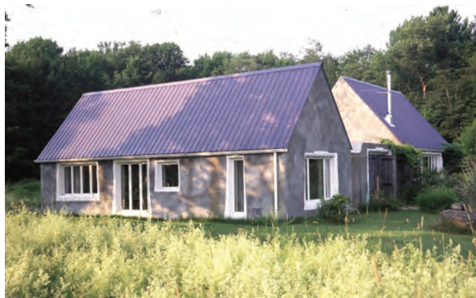
Fig. 7. First permitted strawbale building. A retreat center in Kortright, N.Y., 1989. Finished with gunite.
