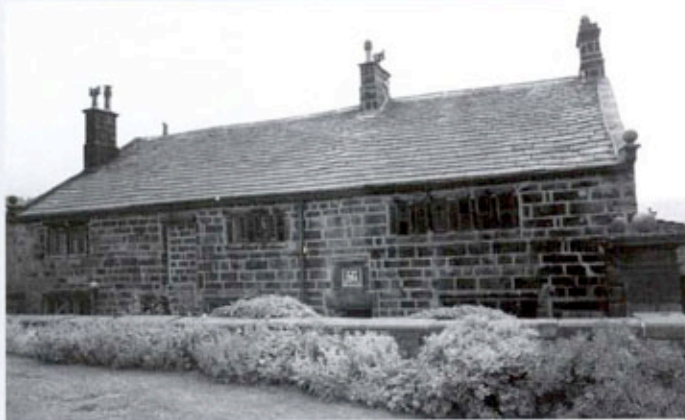
A house built in England in 1759: its original stone-shingled roof is still intact.
