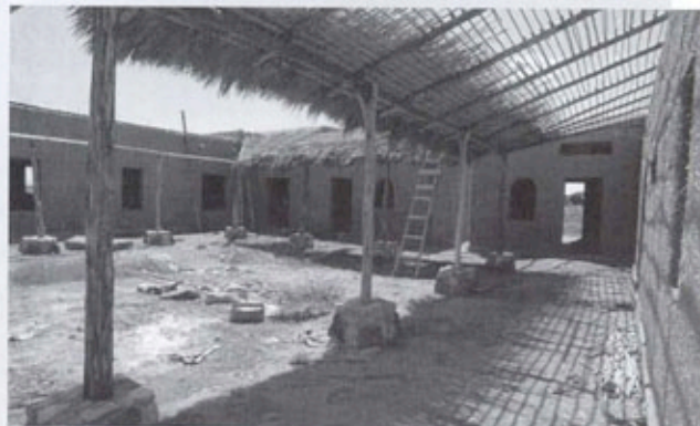
Exterior view of the Save the Children building while under construction, showing straw bale and straw-clay block walls and the construction of the porches using a traditional Mexican palm-thatching technique for the porch roofs.
