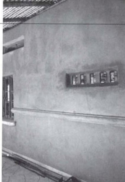
Exterior view of the Save the Children building, showing earthen plaster and the use of gallon jars for windows.
