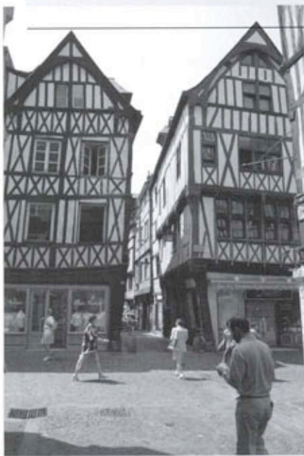
There are hundreds of thousands of houses all over Europe, like these in Rouen, France, that are timber-frame structures with wattle and daub infill finished with lime plaster. These buildings are over 200 years old.
