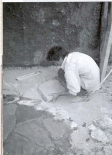
The recycling of used concrete into the floor of a house in Mexico.
