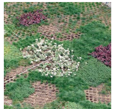
A green roof installed atop Seattle's City Hall in 2003 significantly lowers heat generation and serves as an important component of a rainwater harvesting system that reduces the burden on the municipal water supply and wastewater systems.
