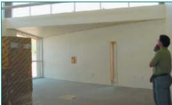
Green Building Inspectors on a job site.
