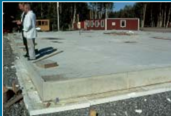
Shopping mall in Trondheim, Norway. Steel columns on insulated spread footings and nonload-bearing walls (grade beams) on FPSFs with insulation on the inner side and under the grade beams. Eliminates the need to protect exterior vertical insulation. Left: Svein Erik Torgersen, Right: Jan Vincent Thue, leading Norwegian FPSF researchers in the early 1970s.
