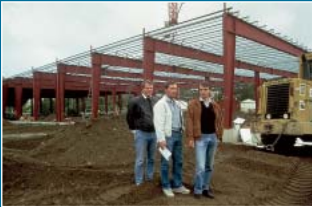
Shopping mall in Trondheim, Norway. Steel columns on insulated spread footings and nonload-bearing walls (grade beams) on FPSFs with insulation on the inner side and under the grade beams. Eliminates the need to protect exterior vertical insulation. Left: Svein Erik Torgersen, Right: Jan Vincent Thue, leading Norwegian FPSF researchers in the early 1970s.
