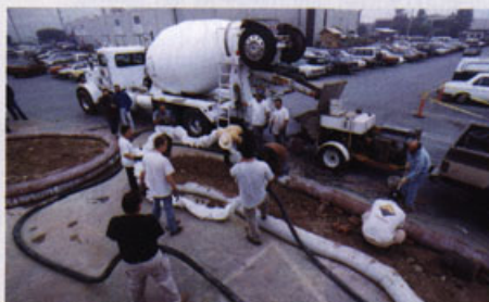
Superadobe/superblock coils under construction, demonstrating pumping method.
