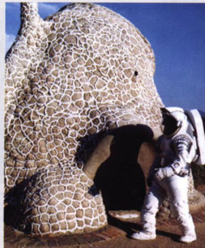
The "Mars One" prototype employed in-situ unstabilized earthen material for construction and testing. Its reptile texture is the result of terrestrial demonstration of a random pattern finish.
