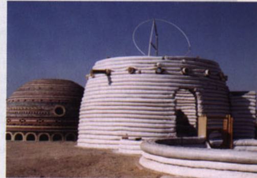
Hesperia Museum and Nature Center utilizes 91 percent in-situ materials to construct stabilized superadobe/superblock coils, with both pumping and manual systems.
