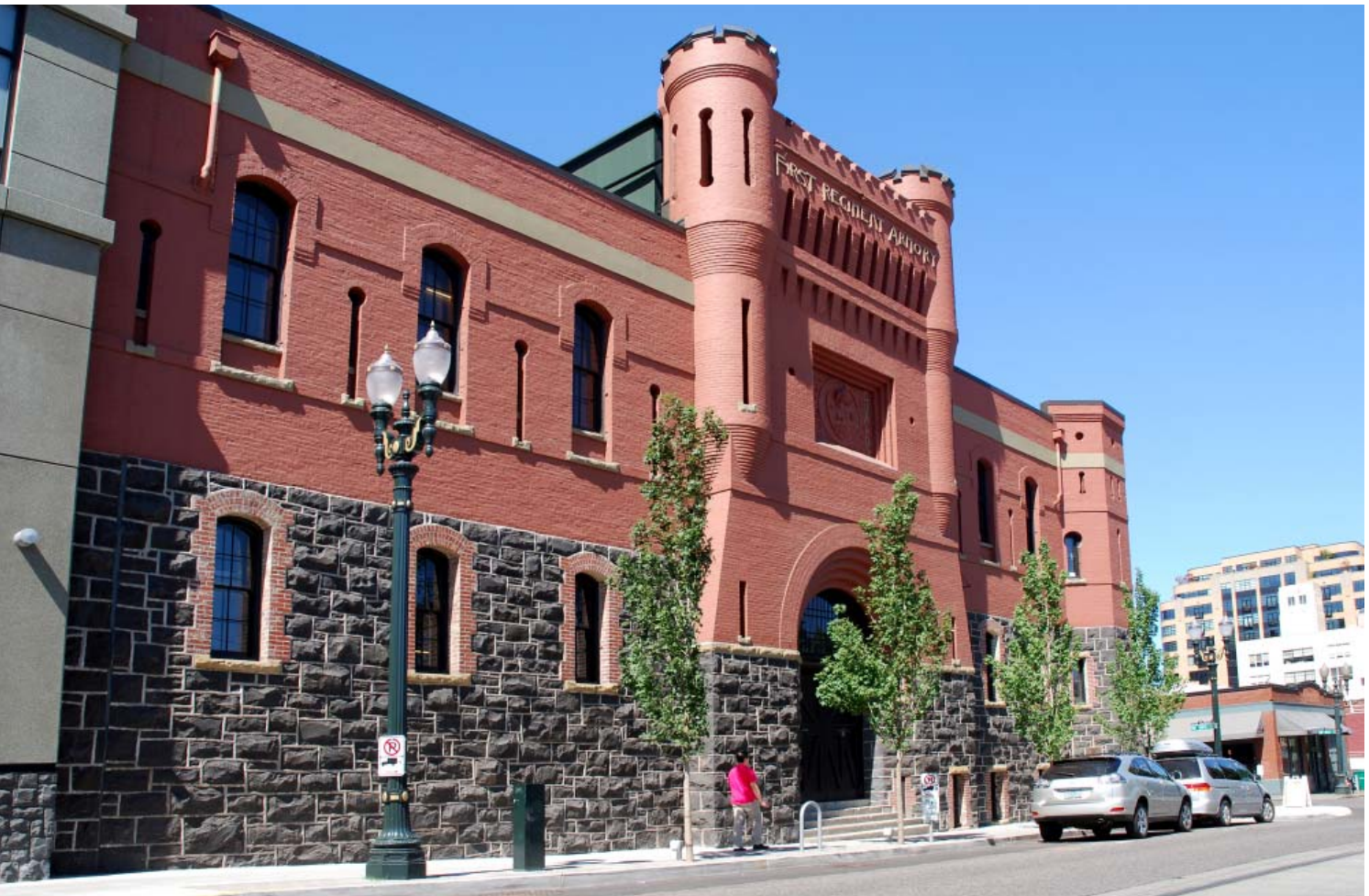
Gerding Theater at the Armory, AIA/COTE 2007 Top Ten Green Projects honorable mention. GBD Architects Inc., Portland, Ore. Photo courtesy of GBD Architects Inc.
