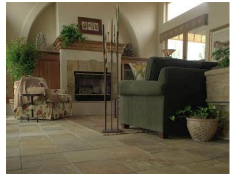
Highly conductive tile is a very effective radiant floor finish
