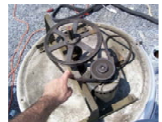
Ventilation fan belt adjustment
