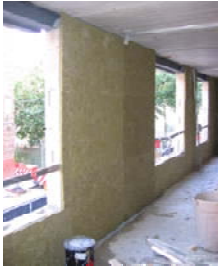
1-inch mineral wool (picture taken prior to steel stud installation)
