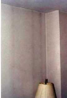
Particle deposition due to thermal bridging
