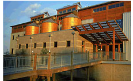
Rainwater catchment system with cisterns at Philip Merrill Environmental Center, Annapolis, Md.
