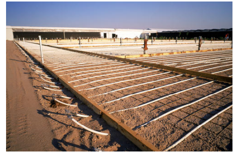
Radiant tubing for a greenhouse before slab is poured.
