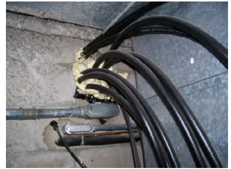
Air sealing at an exterior wall penetration
