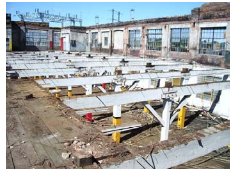
Deconstruction of a building
