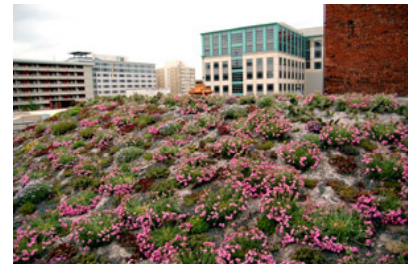
Silene caroliniana plantings on the south side of the ASLA's green roof contribute to the building's overall vegetation strategies.
