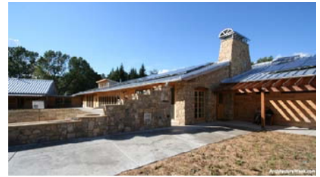
2007 AIA/COTE Award recipient, the Government Canyon Visitor Center, Helotes, Tex., designed by Lake/Flato Architects. This sustainable design minimizes the impact of the building on the land and fragile water resources in this region
