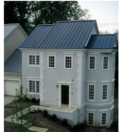
PV roofing system displaced traditional roofing materials
