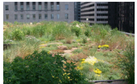
The green roof on Chicago's City Hall, completed in 2001, was designed to test different types of green roof systems, heating and cooling benefits, success rates of native and nonnative vegetation, and reductions in rainwater runoff.
