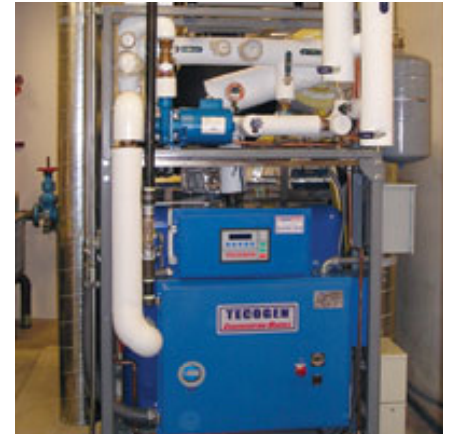
Commercial cogeneration unit
