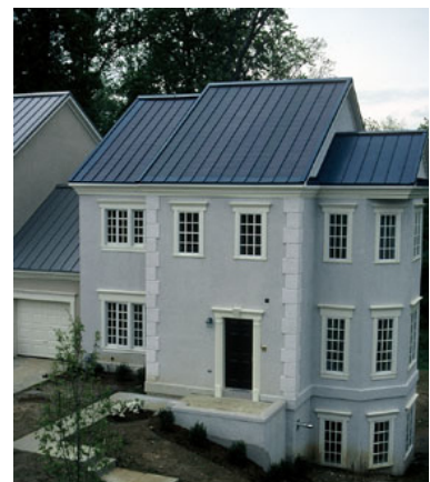
PV roofing system displaced traditional roofing materials
