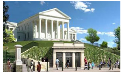
A sensitive restoration and earth-sheltered addition to the Virginia State Capitol Building, designed by RMJM Hillier. The original architect of the Virginia State Capitol was Thomas Jefferson
