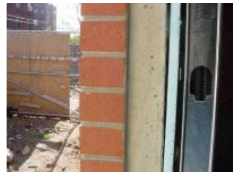
0.5-inch XPS thermal break
