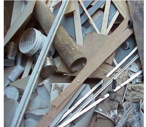
Comingled construction debris
