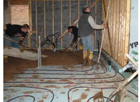
Concrete is poured over radiant tubing and insulation in a home.
