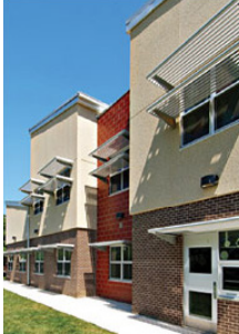
Glebe Elementary School—Arlington, Va., by BeeryRio Architecture + Interiors. Passive solar design strategy incorporated into the exterior of the building (photo courtesy of Loan Pham).
